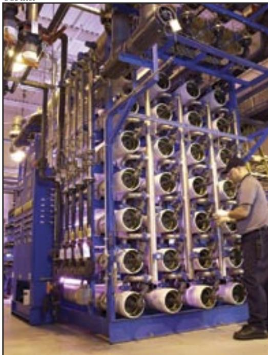
**FIGURE 3.** Reverse osmosis membranes can be cleaned onsite or off-site, depending on your facility's needs. Auditing membrane condition on a regular basis can alert you to other issues within your water-treatment system
