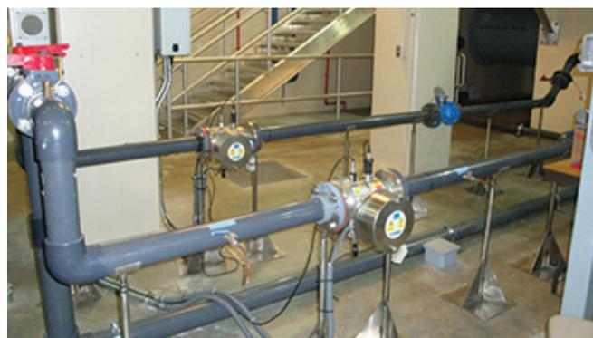
**Figure 1.** ETS-UV™ systems used as part of an AOP pilot study at the Greater Cincinnati Public Water Works
