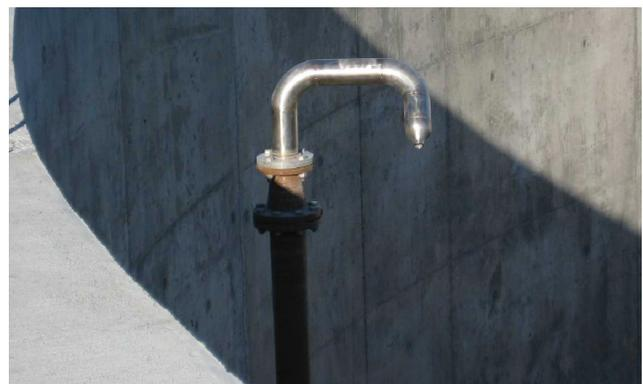
Optional top nozzle for breaking surface crust.
