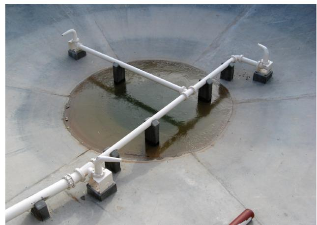
JetMix™ System proprietary nozzle placement.
