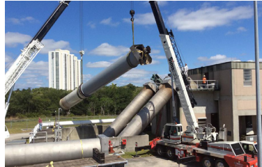
Inspect, repair or replace screw pumps
