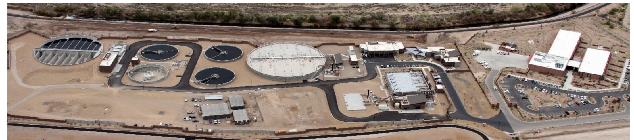
Figure 8. Agua Nueva Water Reclamation Facility, Pima County, Arizona
