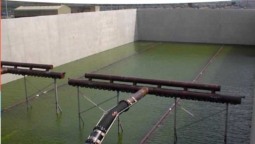
The state-of-the-art design of the Floating Effluent Decanter does not utilize electro-mechanical equipment in the basin.
