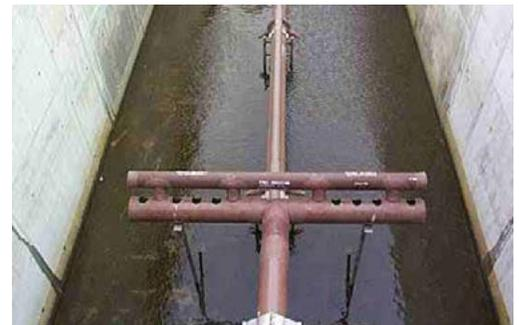
Supernatant Decanters do not include spring loaded valves and liquid can be drawn closer to the surface if needed.
