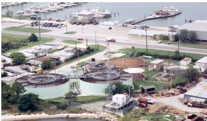
Biological Nutrient Removal Process 1 MGD Installation in Alabama
