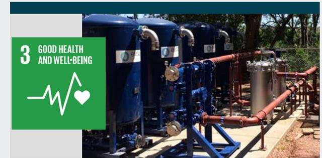
**Recovery of potable water from a PFOA contaminated well in Stratmoor Hills**
